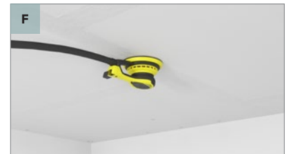
Sand joints: After sanding with preferred tool, ensure that the joints are perfectly smooth.
