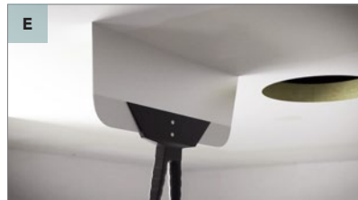
Check joints and center of panels.
